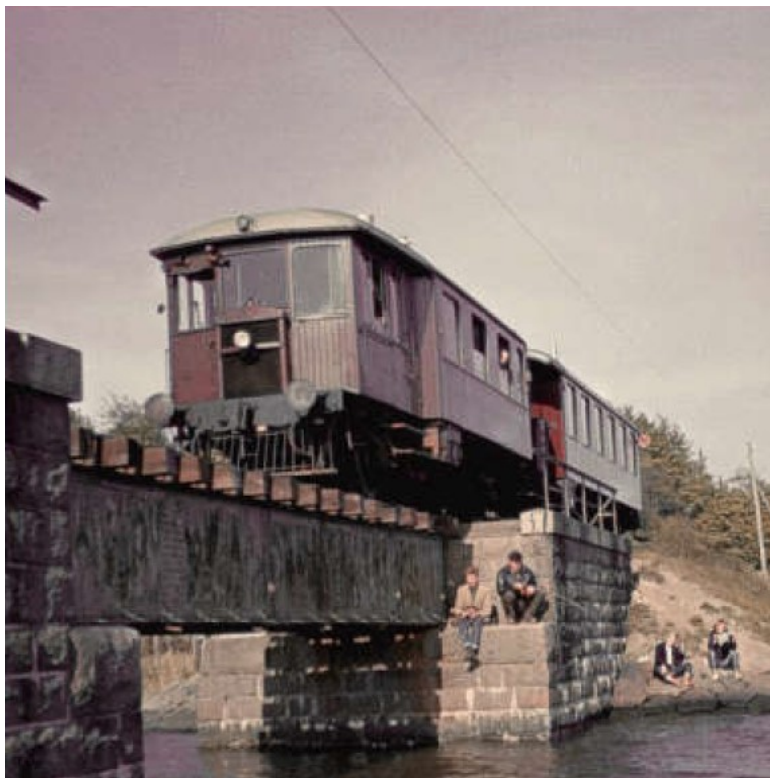
Broen i original tilstand.
