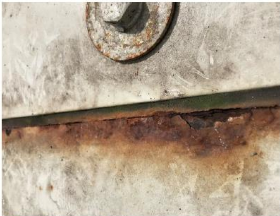
Figur 9: Korrosion langs gummifuge
