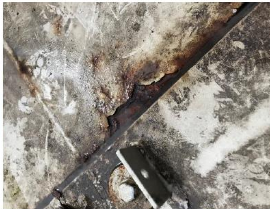
Figur 10: Korrosion langs gummifuge
